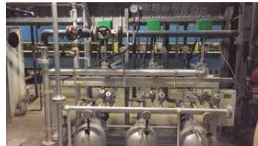
Less energy loss thanks to the new condensate lift station in Moudon
