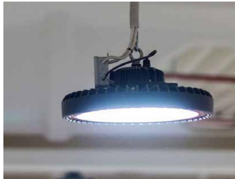
Controllable LED lights adjust brightness according to the level of daylight
