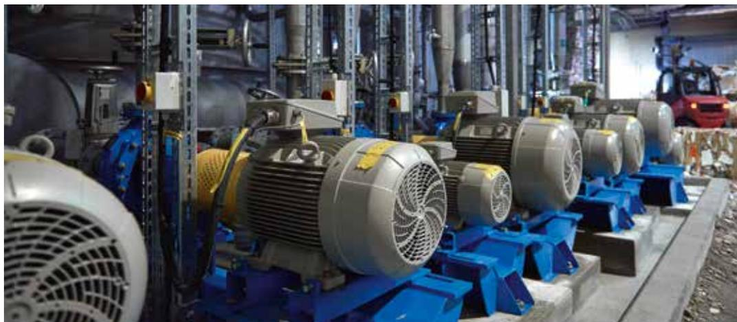
Andritz pumps driven by Siemens motors on the 120m<sup>3</sup> clarified water tank
